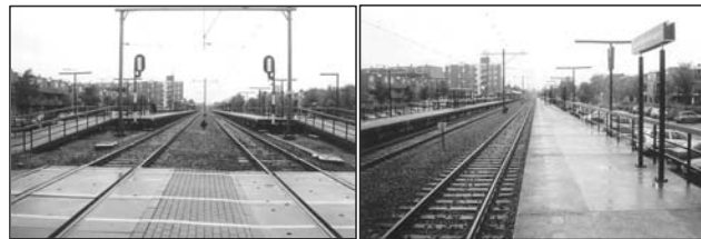
Concrete infrastructure of Hoorn-Kersenboogerd station
